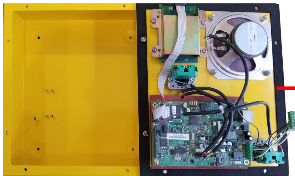
The faceplate is mounted inverted on the side of the enclosure
