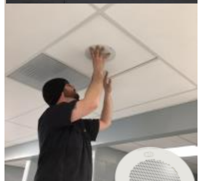
011121 Auxiliary Analog Speaker, daisy chained off of SIP Speaker
